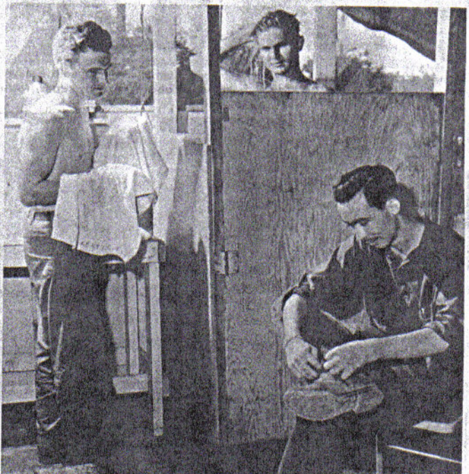
No, this isn't Stateside. It's the interior of a Seabee tent on Guam. The wash stand and shower bath were made out of Jap cement and piping
