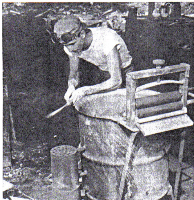
Built of salvaged Jap material, this washing machine boasts an unusual feature. Heater and core boiler keep water at constant temperature
