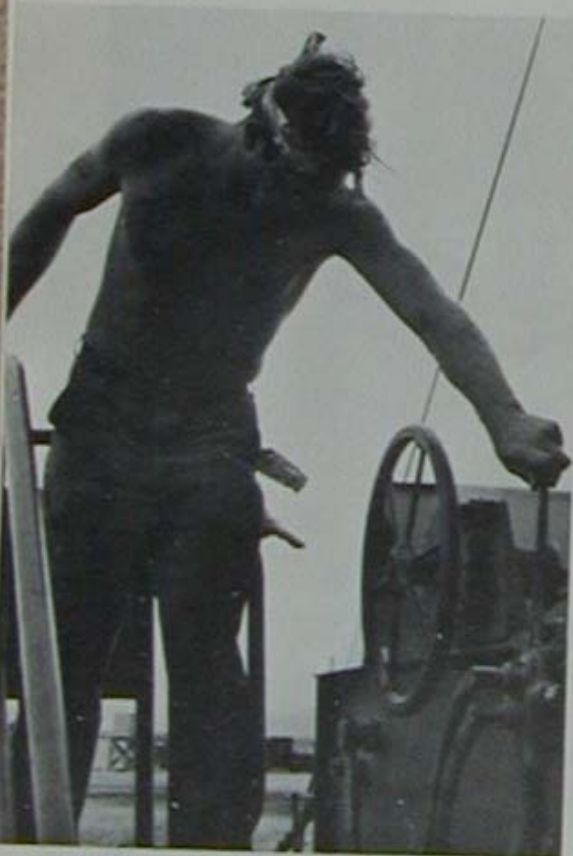
E02 Richard Reda pulls the lever that releases the asphalt into dump trucks below.
