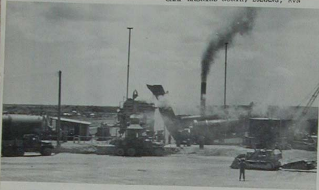
The asphalt plant in operation.
