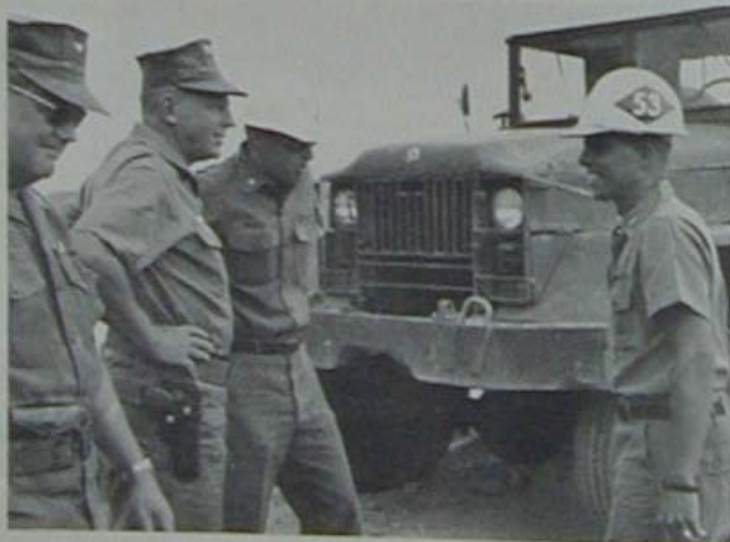
RADM E.P. Bonner (second from left), Commander NSA Da Nang, talks with LT J.B. Green, Officer-in-Charge of MCB-53's Lang Co bridge project. Looking on are CAPT J. E. Powell (left), Commander 30th NCR, and CDR R.K. Miller (third from left).
