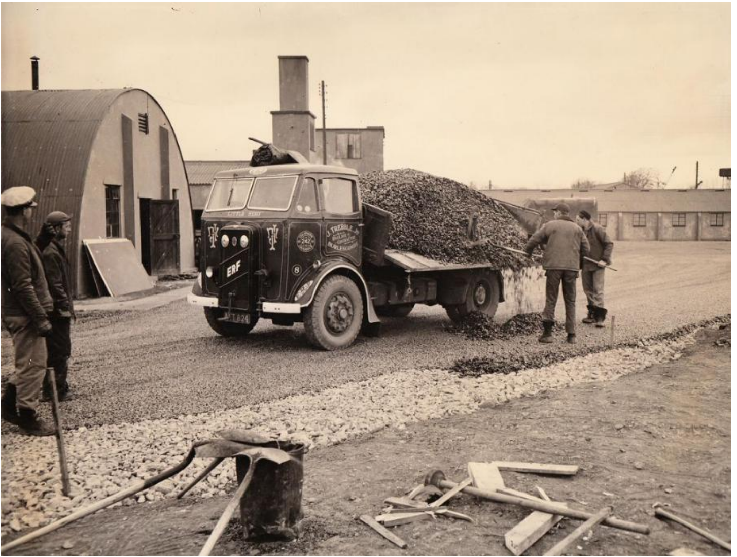
Seabees use a rare English side dump truck for road construction in February 1945. (U.S. Navy Seabee Museum photo)
