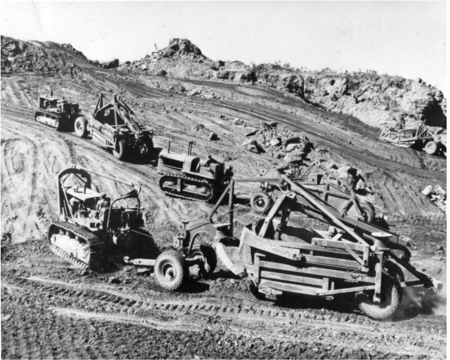
Seabees with the 62nd Naval Construction Battalion work around the clock to build an airstrip and camp areas on Iwo Jima in March 1945. (U.S. Navy Seabee Museum photo)
