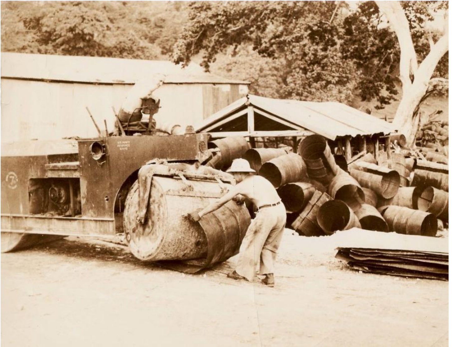
Seabees with the 7th Naval Construction Battalion make roofing tiles from old oil drums in January 1945. (U.S. Navy Seabee Museum photo)
