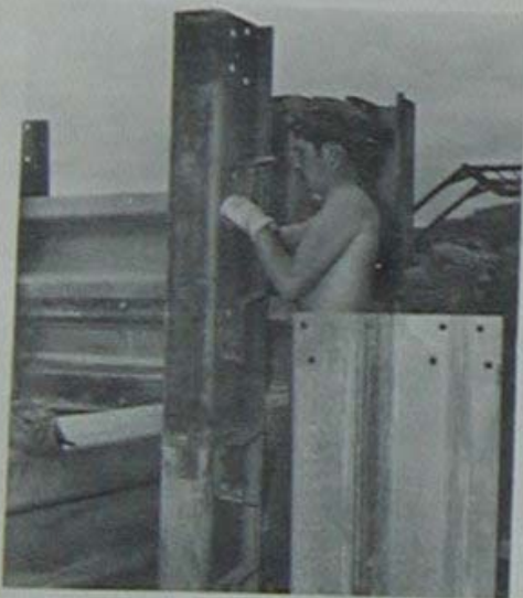
BU3 Richard Boyce (center) from Newcastle, Delaware, and SW2 Bill Ward (background) from Harrisburg, Pennsylvania, tighten down revetment brackets during the construction of a computer facility.
