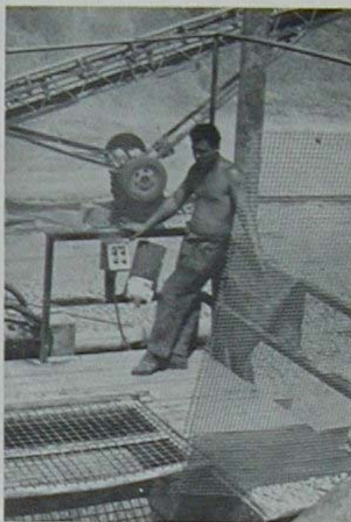
E02 L. F. Drinkwine from Willsboro, New York, operates the rock crusher at Vinh Dai.
