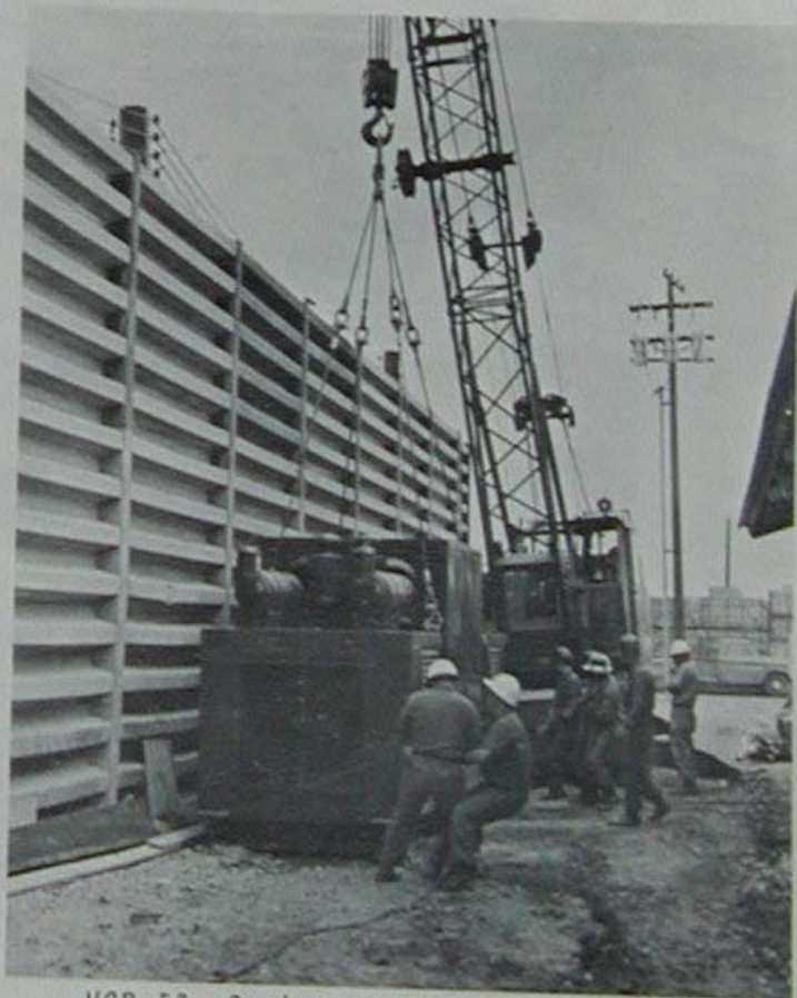
MCB-53 Seabees, with the aid of a crane, put a generator in place that will be used for the Data Processing facility.
