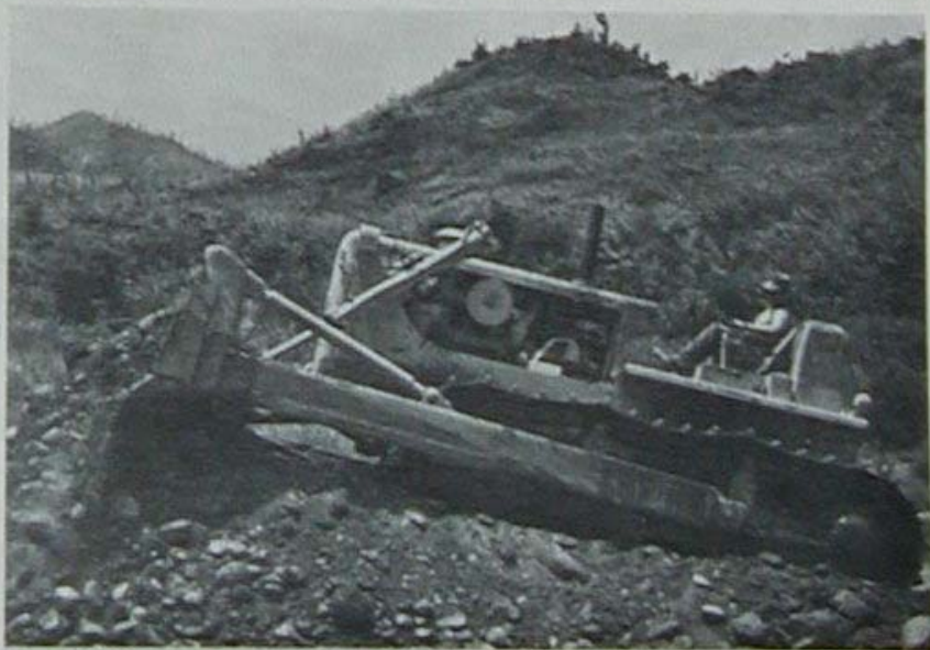
Piling up rock at the Quarry site is E01 J.R. Oswalt from Weaver, Alabama. The rock is then loaded into dump trucks and taken to the base camp at Vinh Dai to be crushed.
