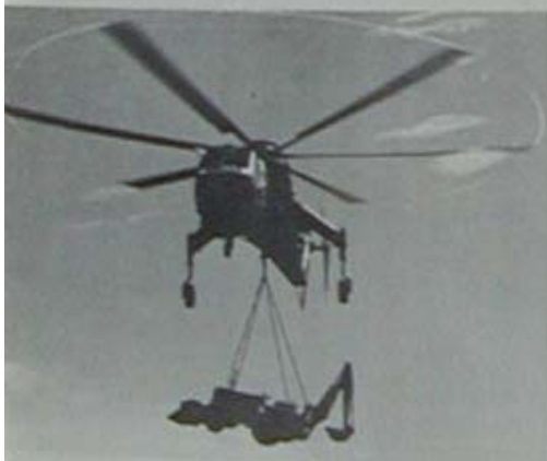
A CH-47 Sky-crane arrives with a miniature backhoe hooked beneath it.
