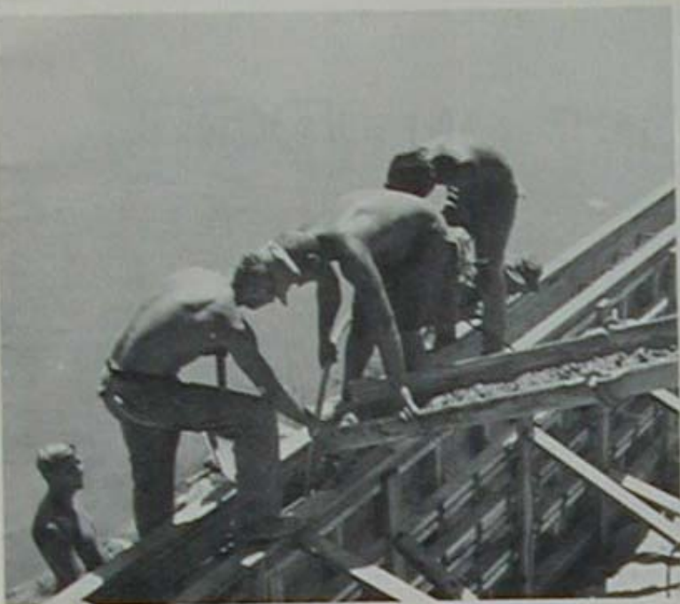
Builders pour a head wall during the early stages of construction.
