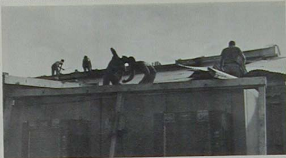
Foxtrot Company personnel repair damage done to the galley roof.
