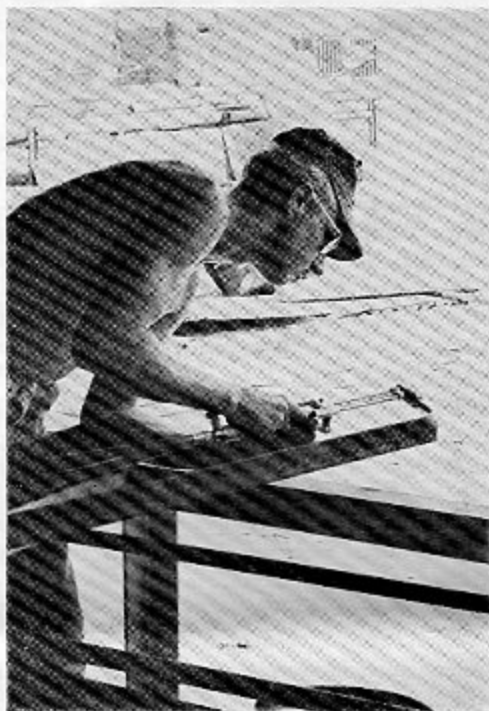
SWE2 Gerald GROON, "D" Co., from Akron, Iowa, cutting angle iron with cutting torch.
