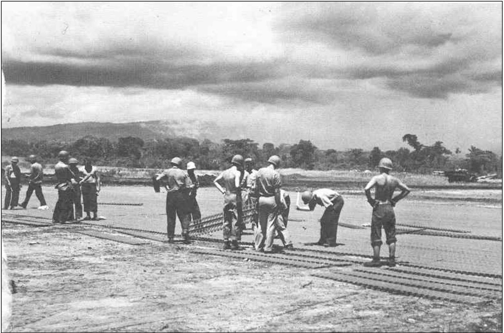
Repairing Marston mat at Henderson Field, Guadalcanal
