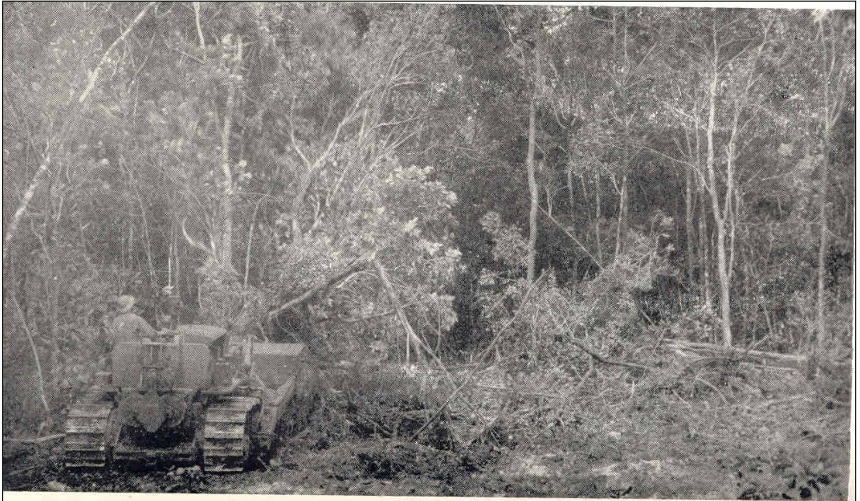
Here are six views showing the evolution of a jungle airfield. 1. Clearing operations – first day. (Official U. S. Navy Photo)
