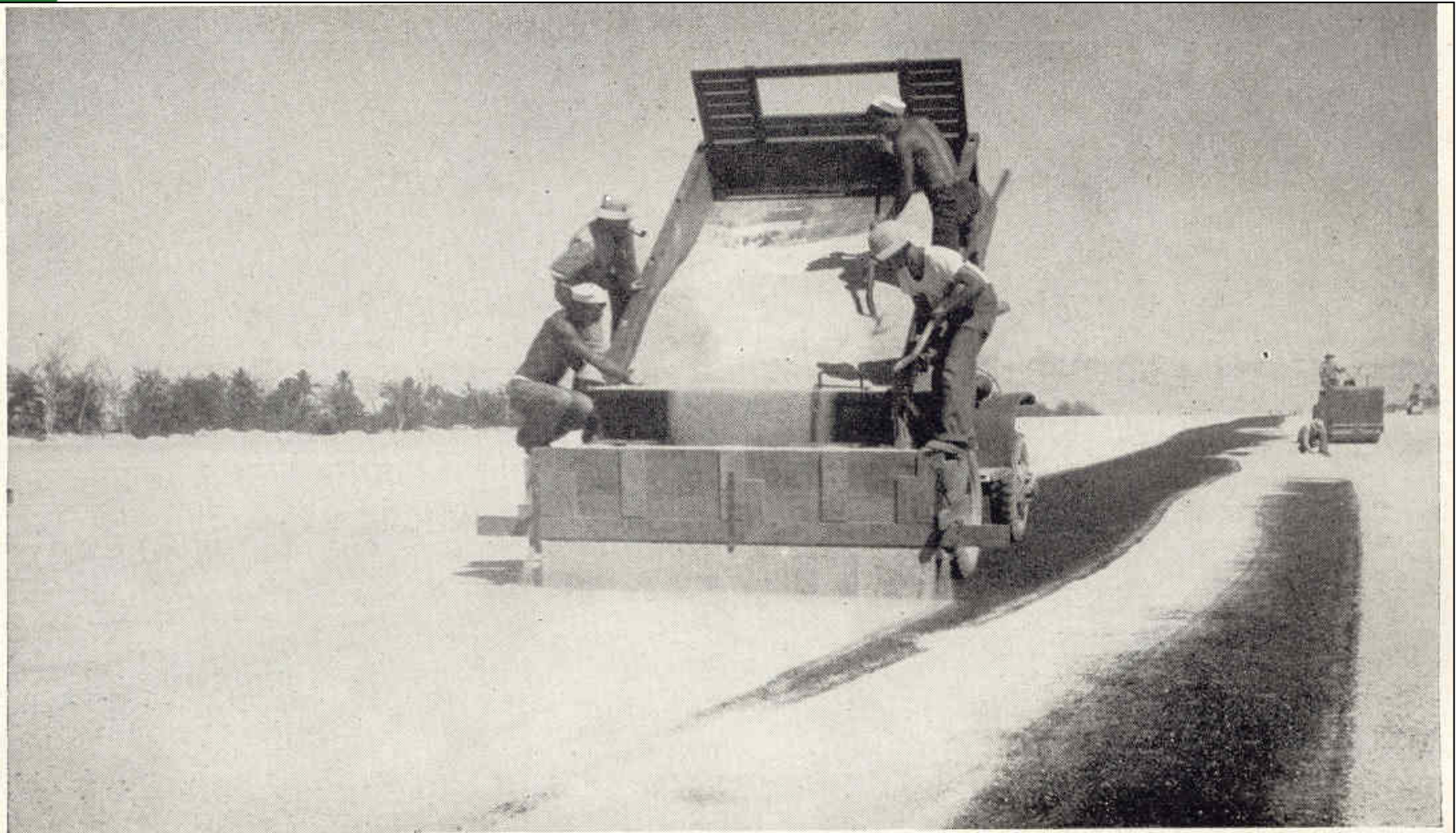
5. Surfacing with finely crushed coral – twelfth day.
