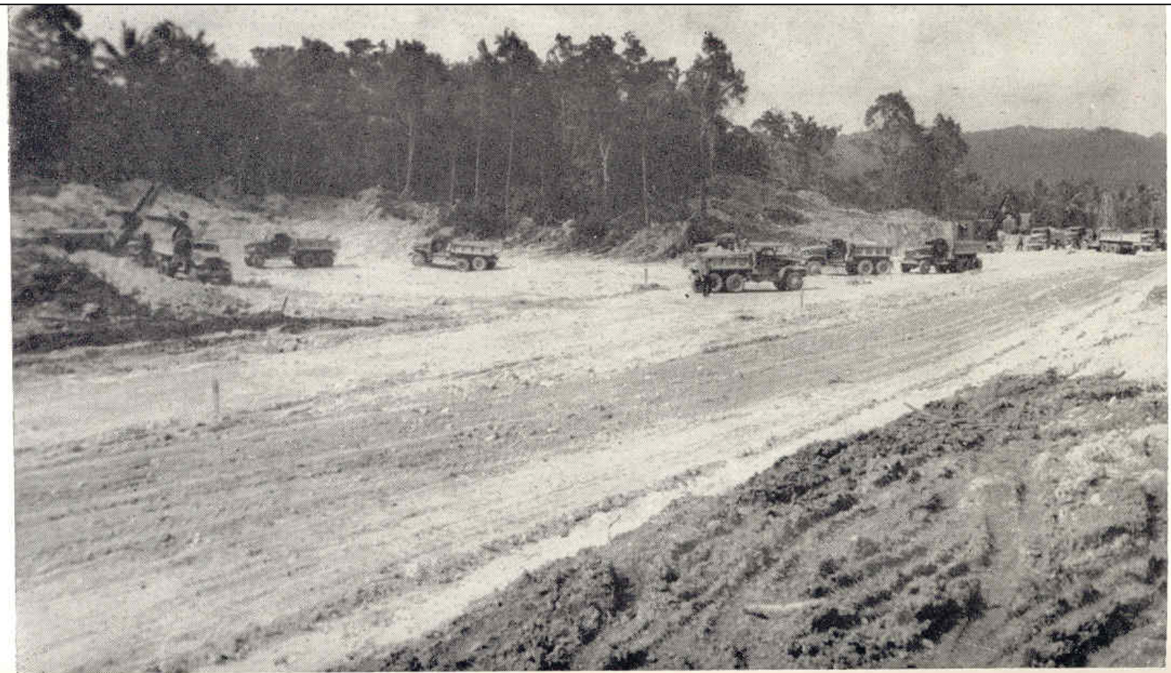
3. Excavating hardstands — parking areas — sixth day.
