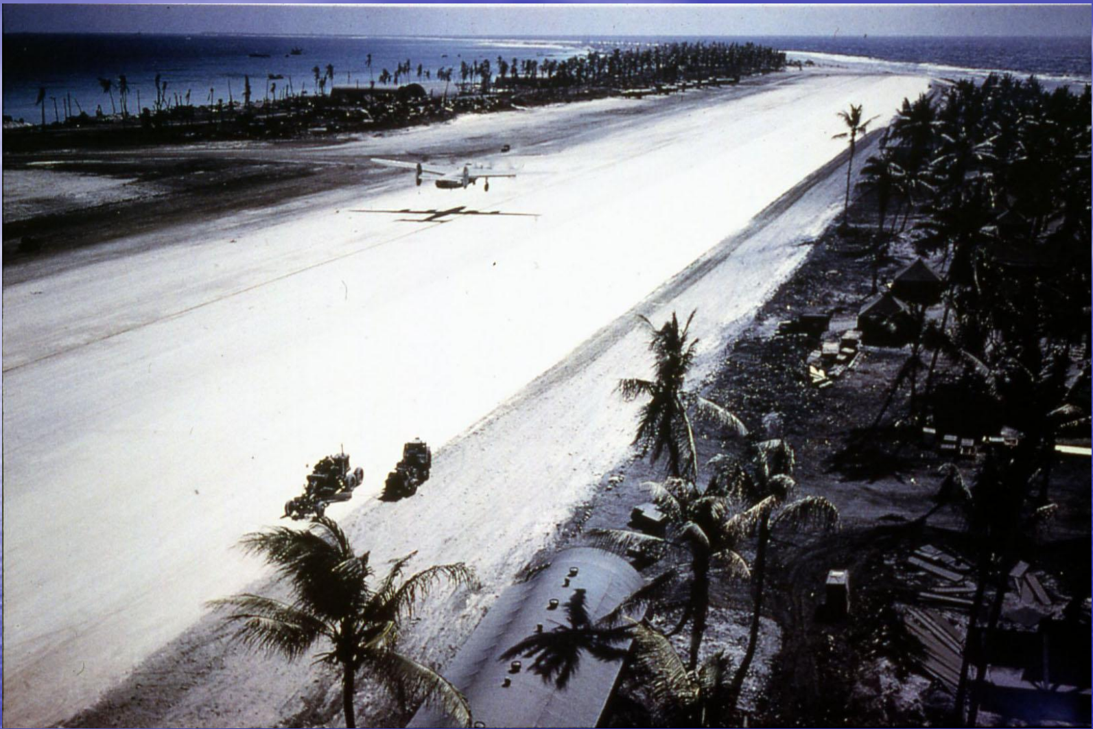
New coral runway supporting long range Army Air Corps B-24 bombers on the new airstrip at Munda, in the Solomon Islands
