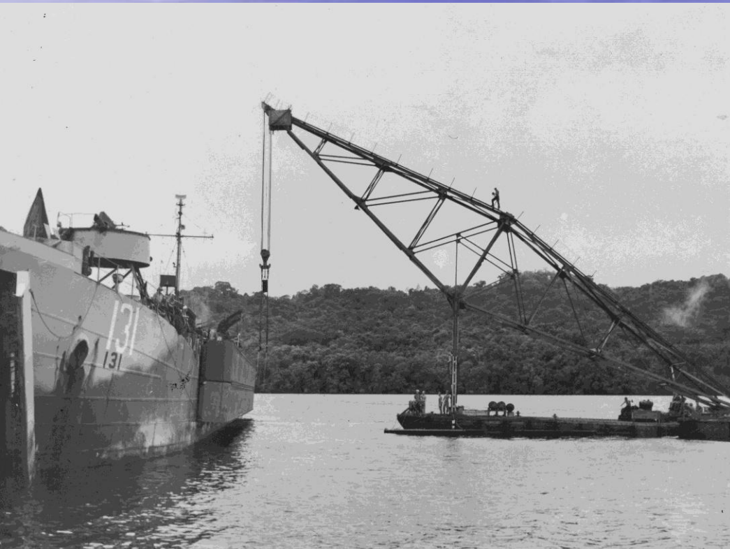
A 60-ton crane on a pontoon barge, is hoisting a pontoon causeway to lash it to the side of an LST.
