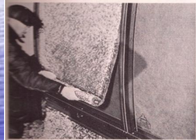
FASTENING INTO CHANNEL
