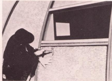
NAILING TO WINDOW SILL
