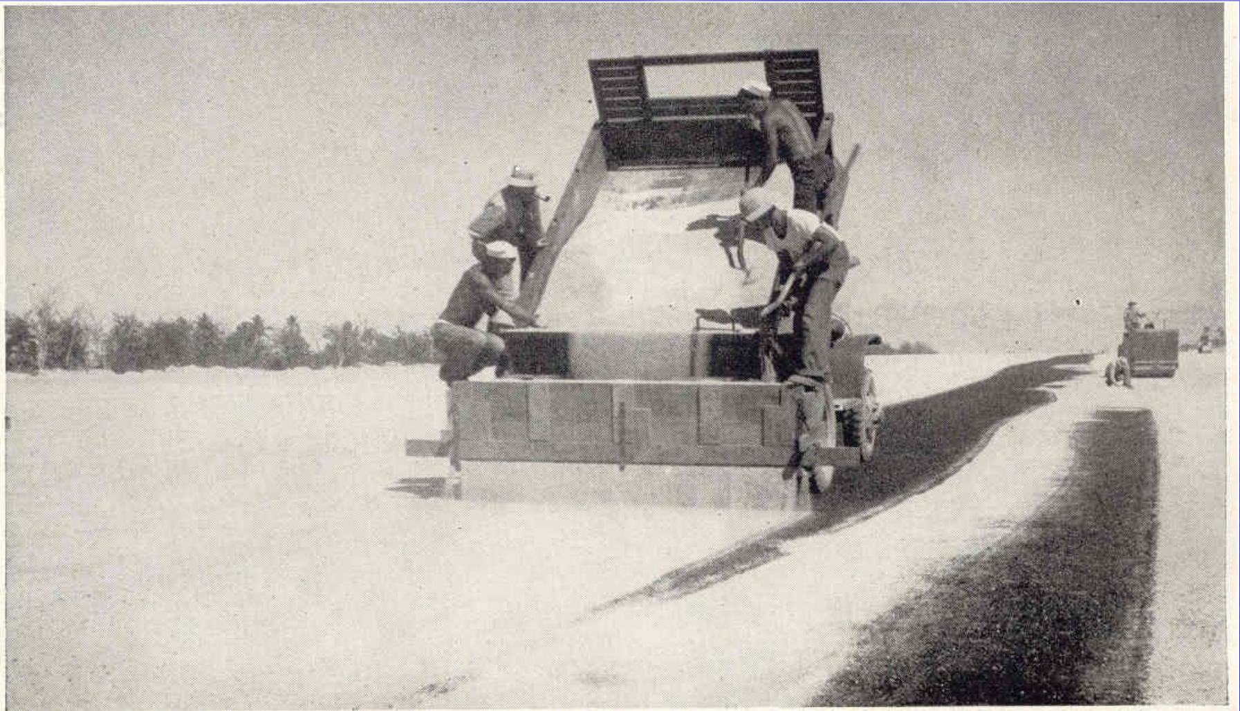
5. Surfacing with finely crushed coral – twelfth day.
