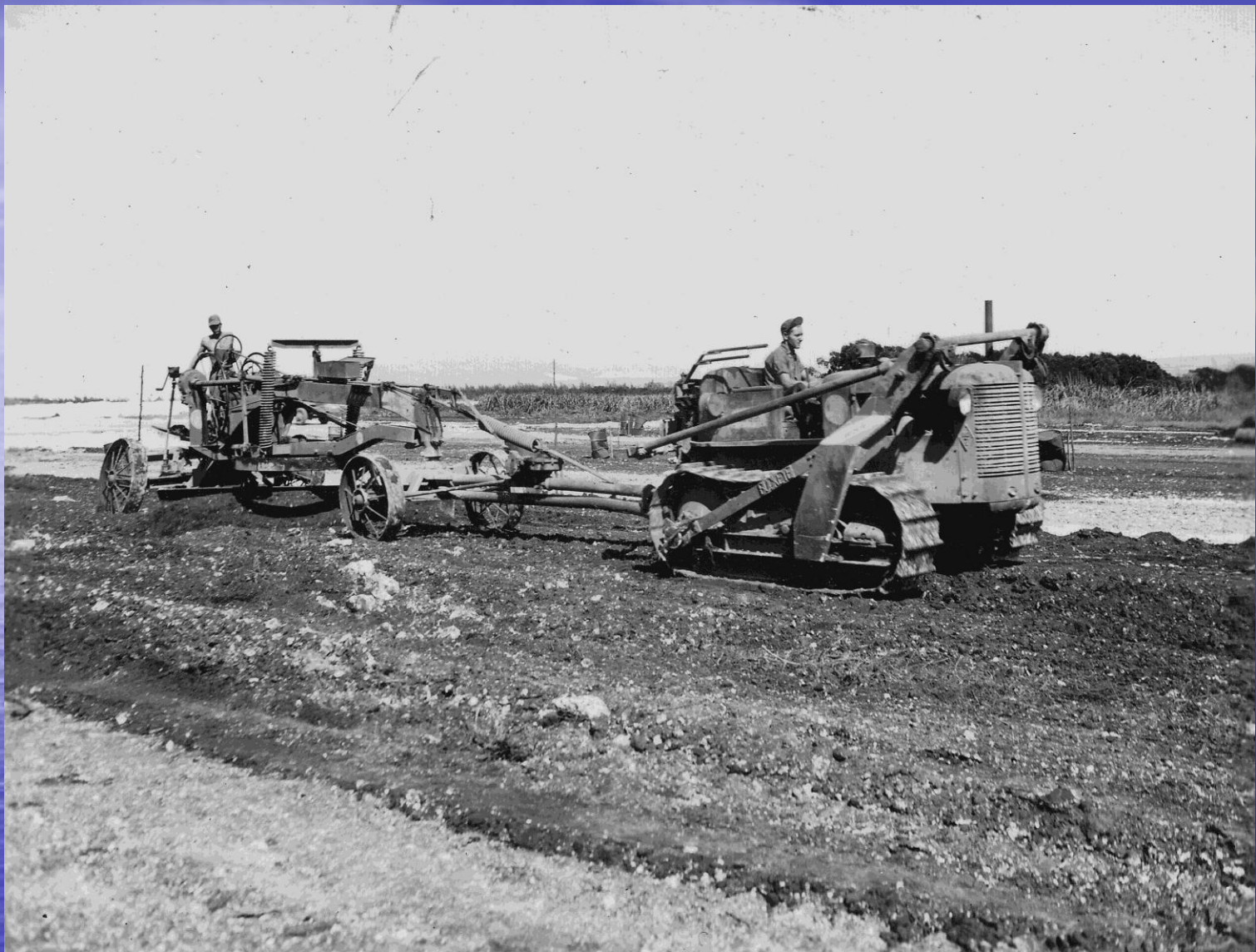
Old Massey-Ferguson grader being pulled by an Allis-Chalmers tractor in January 1945 on Tinian, by the 135 th NCB.
