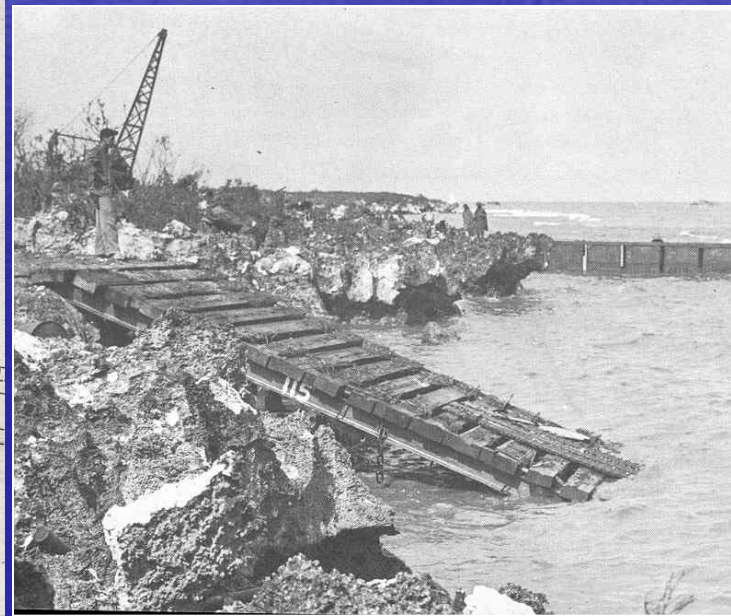
The flexible timber treadway was laid in place by retracting the Amtrac, as shown at left
