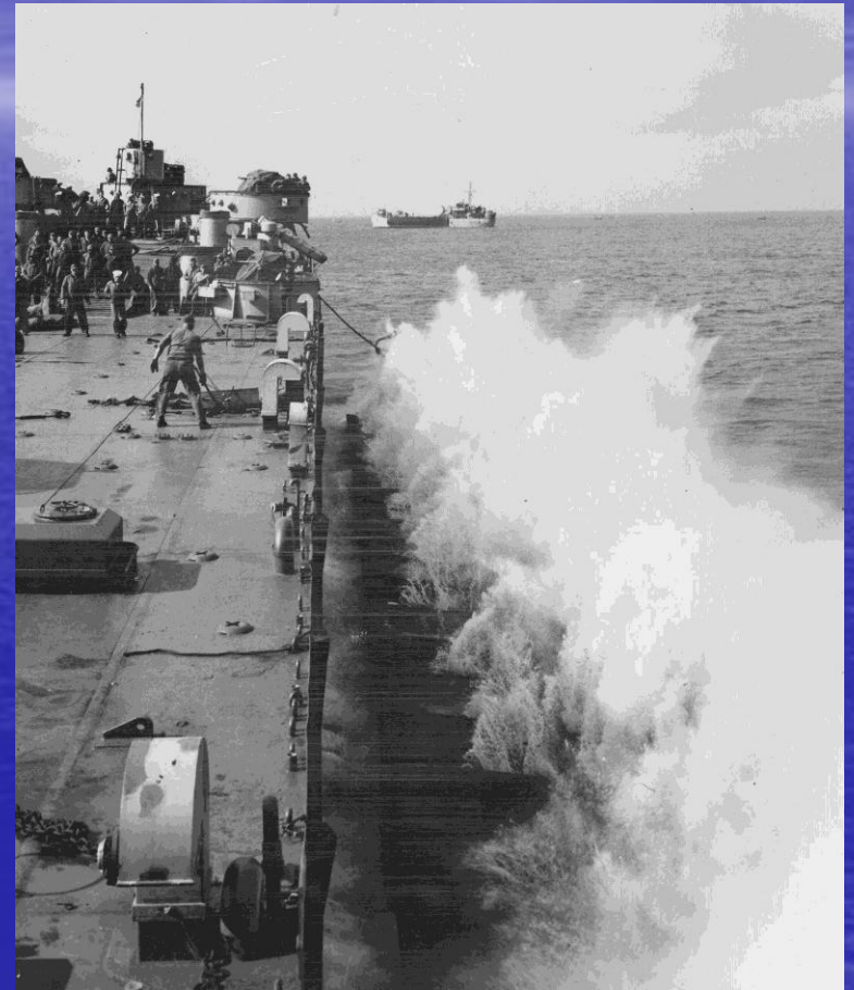
Cutting a pontoon causeway loose from the starboard side of an LST, prior to deployment at the beachhead
