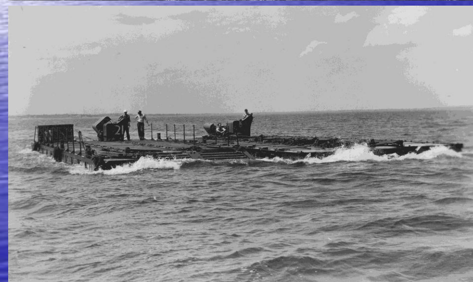
6 x 12 pontoon seaplane barge underway, without seaplane. Note ramp at one end.
