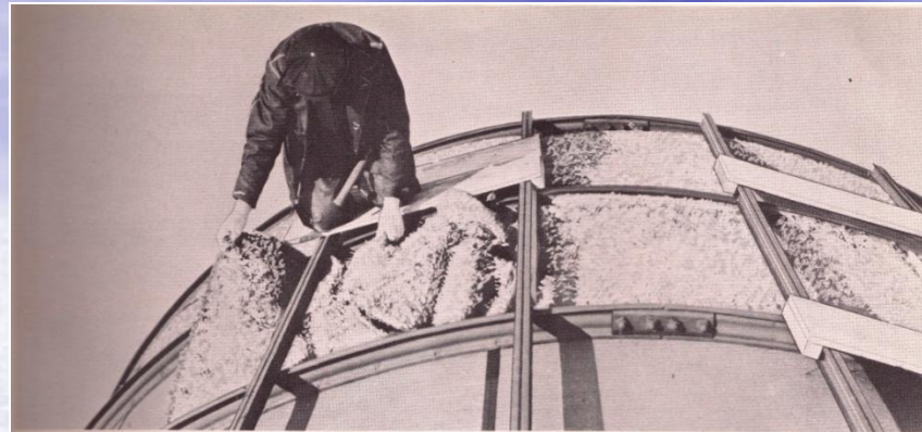
INSULATION APPLIED OVER MASONITE
