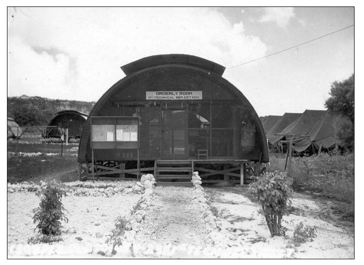
Tropical Quonset 20 with its noticeable 'umbrella hood,' occupied by elements of the 509th Composite Group on Tinian in 1945. Tropical Quonsets employed screened end walls, raised roofs, and additional vent flaps along their sides to promote better air circulation. Note elevation of floor in this example, well above the ground. This enhanced better cooling as well.
