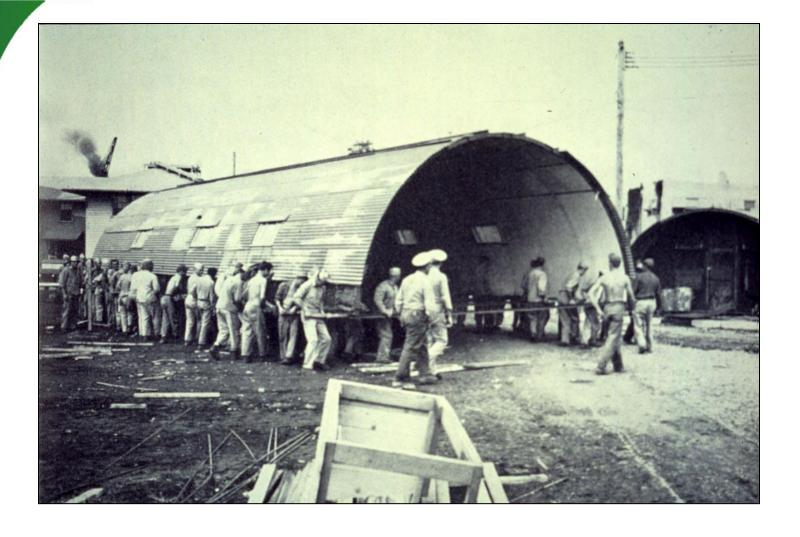
Several dozen Seabees of NCB 90 man-handle a 20 by 48 Quonset Hut on Iwo Jima using steel stretchers with pipe handles, moving it to a new location. An empty Q20 hut weighed about 7000 lbs
