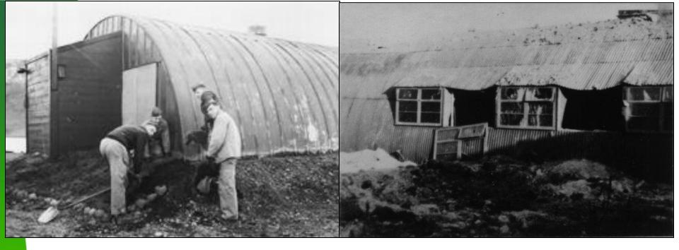
Left - In order to provide additional weatherproofing and insulation for their older style Nissan Huts in Iceland in 1941, American Marines stacked sod around the foundations and tied down the tin roofs with barbed wire. Note the wood frame wind-baffle vestibules, tacked onto the end of the Hut.
