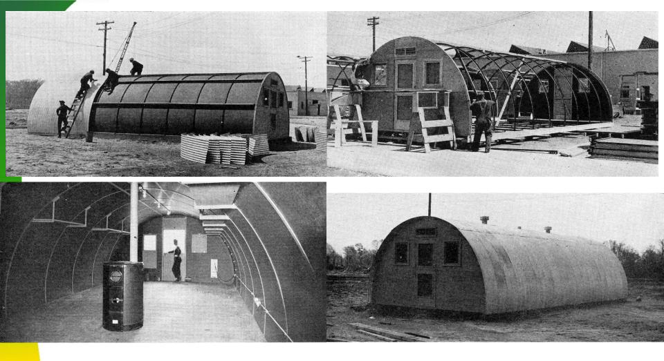
Details of the original Fuller-built 16' x 36' Quonset Huts, assembled at West Davisville in the summer of 1941. The American hut employed masonite interior walls with a galvanized steel shell, and the gap filled with insulation.
