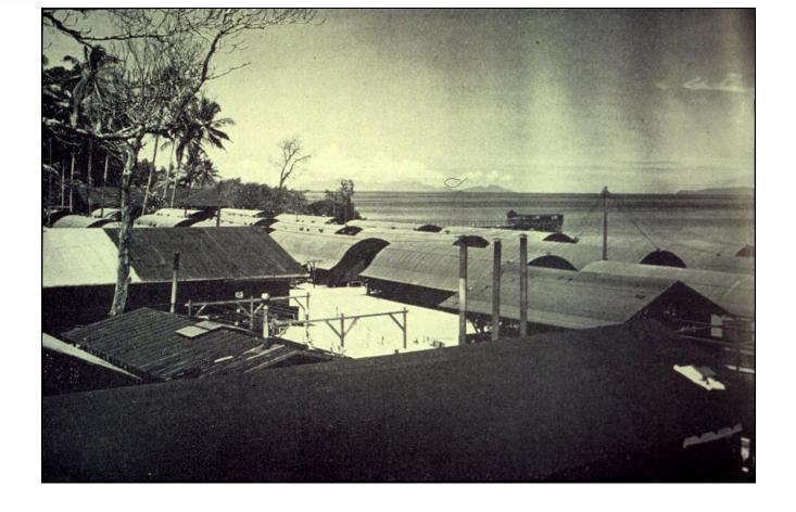
From mid-1943 onward, virtually all of the standard Quonset 20s were modified during construction with open, upturned sides to make them more bearable in tropical climates. This shows the living quarters at Carter City on Florida Island in the Solomons. Frame structures in foreground are the base laundry and one of the power plants.
