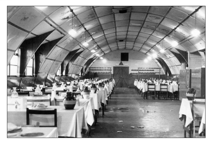
Interior of a 36 ft wide Nissen Hut serving as the officer's mess for the 401<sup>st</sup> Bombardment Group (H) at Deenethorpe Air Base in Northamptonshire, about 100 miles north of London. Note concrete slab floor, window dormers and layout of circular frames (3 ft on center) and connecting purlins. The 401st took this base over from the RAF in November 1943 and remained until June 1945.
