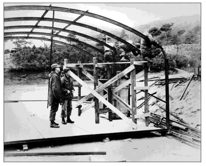
As the US presence in South Korea continued after the 1953 armistice, more permanent facilities were constructed each year. This shows Army Engineers erecting the frames of a post-war straight-side Hut in Korea, sometime after their introduction, in 1954. This modification made more efficient use of the interior floor space.
