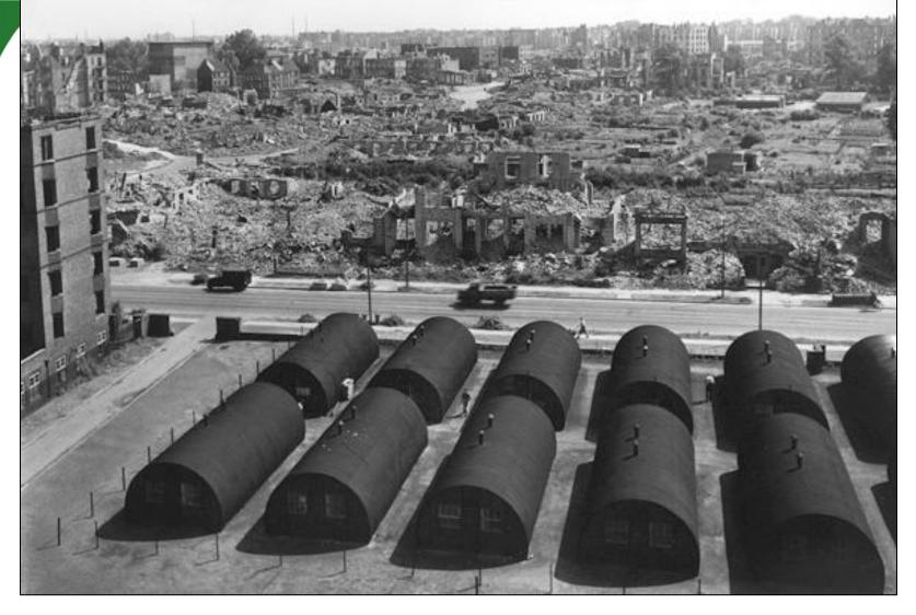
English Nissen Huts assembled in Hamburg, Germany as temporary housing because so many structures had been destroyed by Allied bombing, as seen in 1946. The exterior of these huts were painted with coal tar to enhance solar heat absorption during the cold winter months and better resist corrosion.
