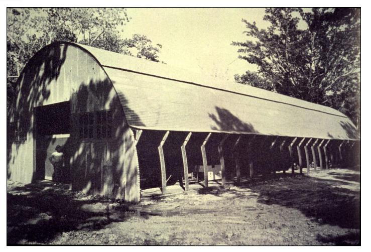
Quonset 40-by-100s were used as warehouses, machine shops, power and pump plant enclosures, etc. Note the large doorway in the end wall. The suffocating heat of the tropics soon led to onsite adaptations, such as that shown here. This allowed better ventilation while keeping most of the rain off of equipment. This shows a refrigerator warehouse at Havannah Harbor on Efate in the New Hebrides.
