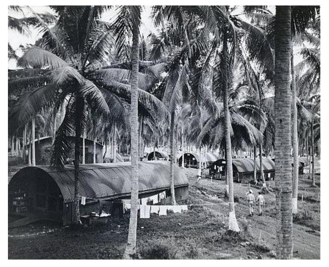
In late 1942 the standard Q20 hut was re-designed with straight sides to better utilize floor space, but these required additional cargo space, so the Navy reverted to the hemispherical design.
