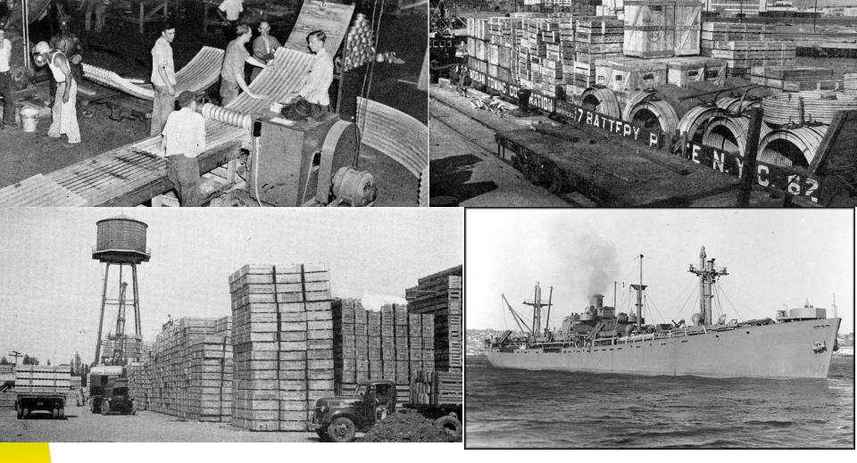
The corrugated steel shapes were bent at Fuller's factory in West Davisville (upper left), and shipped in 12 crate sets, shown at upper right and lower left. Various packing schemes evolved during the war, to make more efficient use of cargo hold space aboard transport ships (lower right.)
