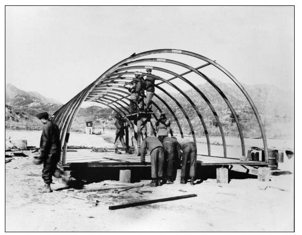
The Korean Armistice in June 1953 necessitated the construction of more permanent military bases south of the Demilitarized Zone (DMZ) for American and Korean security forces guarding the border. This shows a standard 20-by-48 hut being erected by Combat UMR Engineers of the US 8<sup>th</sup> Army.
