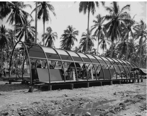
The assembly instructions directed that the Masonite lining be installed first, followed by the wood fiber insulation, then by the exterior corrugated steel sheathing. Image at right shows window and door frames/dormers on a standard 20-by-48 ft Quonset Hut, produced by Stran-Steel
