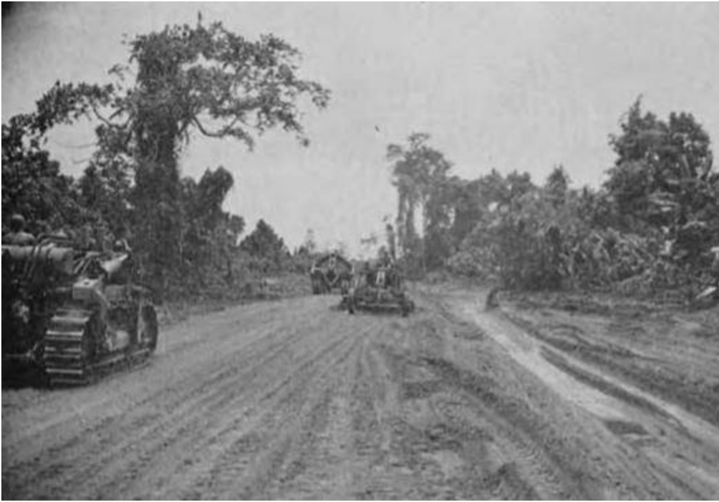
"Marine Drive" nears completion
