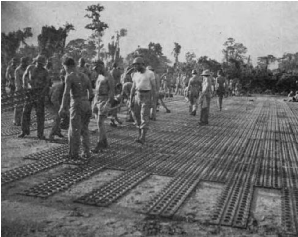
Laying down Marston matting
