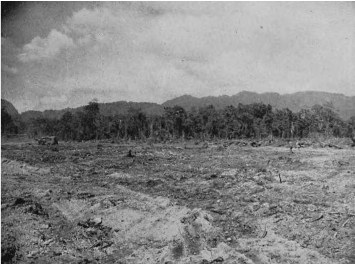
Clearing of the jungle for the Torokina Point Airfield
