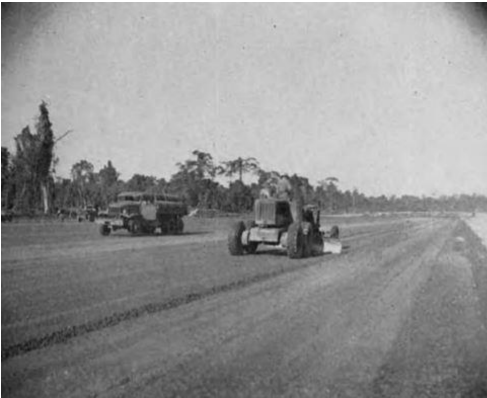
Grading the aircraft apron
