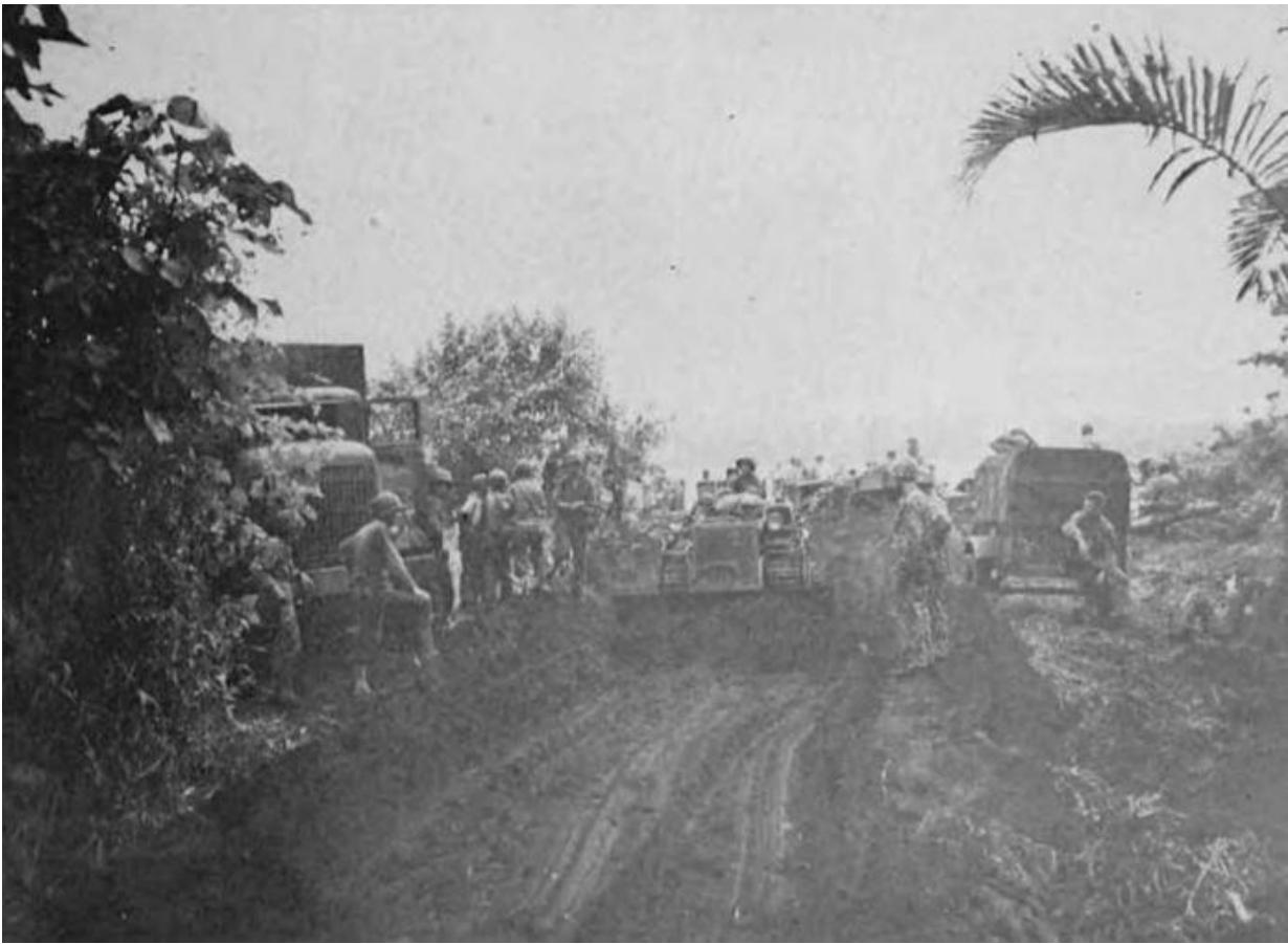
Clearing a path off the beach for the Marines
