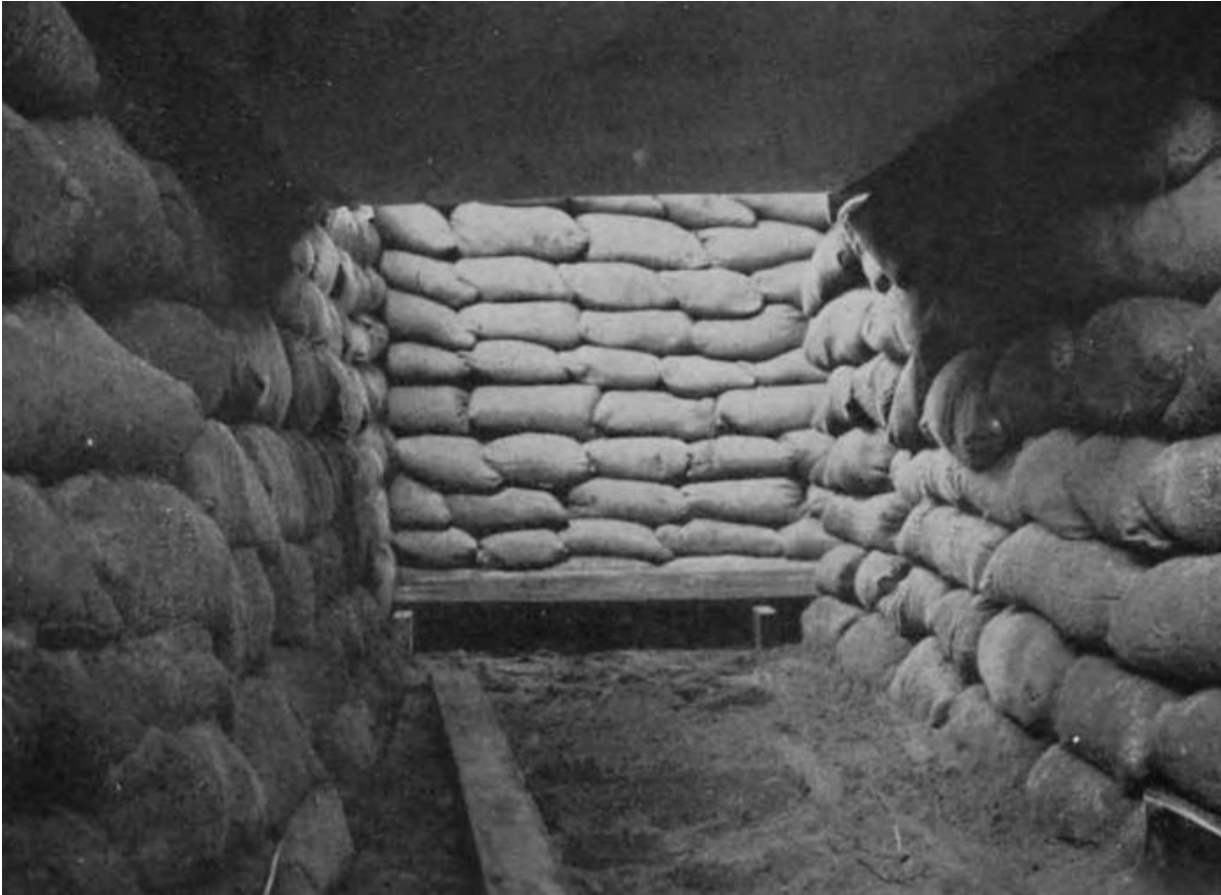
Air shelter for Admiral Halsey, Commander South Pacific Area, built by the 53rd Seabees
