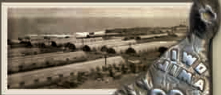
Above: Hospital built on Iwo Jima by the Seabees.
